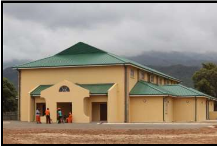
Moshate Community Hall
